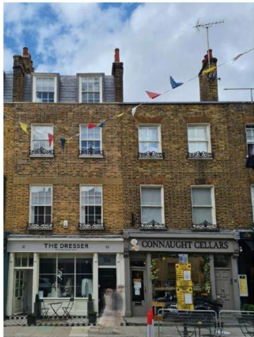
Existing shopfront at 8, Porchester Place (Connaught Cellars)
